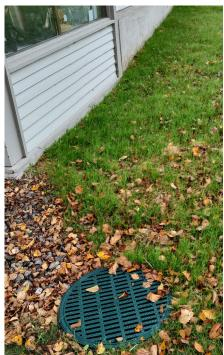
This drain is located on the exterior corner of the Thrift Shop. We recently excavated the pipe leading to this drain because the pipe was crushed and no longer carried ground water away from the building. A new pipe was installed and the system is back in operation, eliminating an odor that had been noticed over many months.
